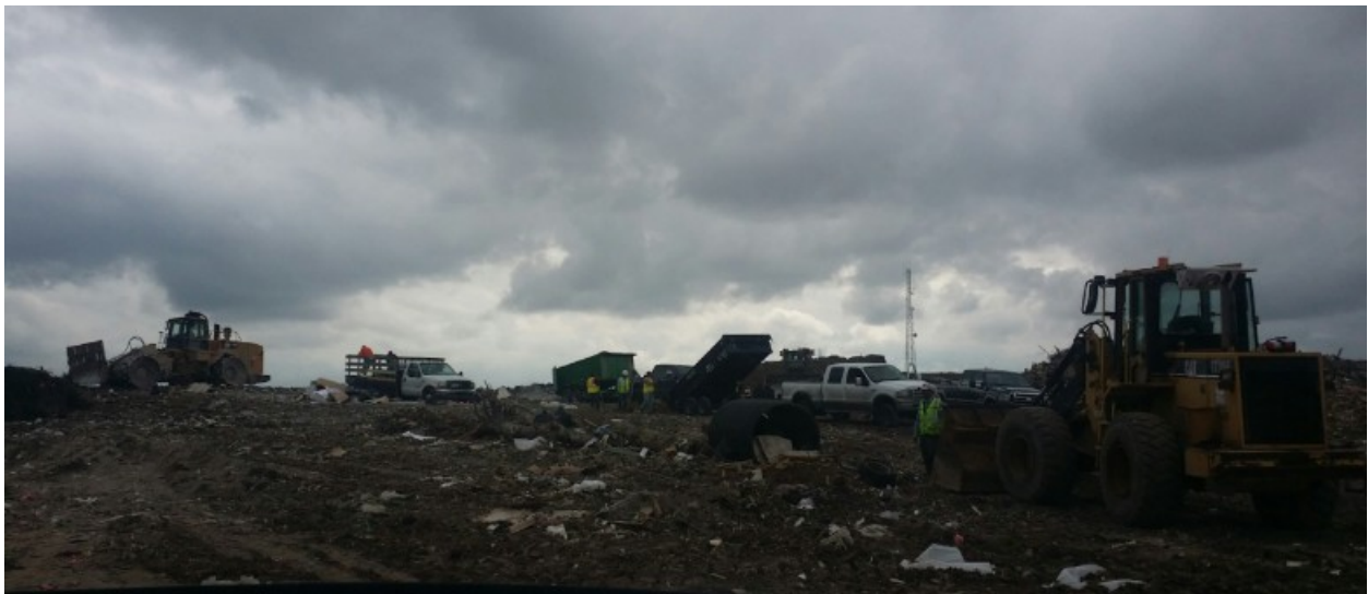
Waste and trash being compacted
